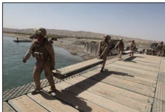
US Marines construct a bridge in Helmand province (ISAF Photo)
