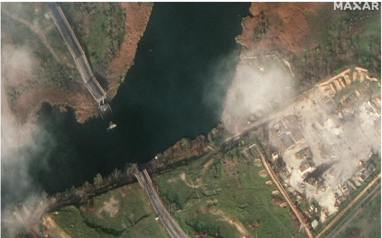
Overview of damage to the Darivka Bridge on November 11. Source: Satellite image ©2022 Maxar Technologies
