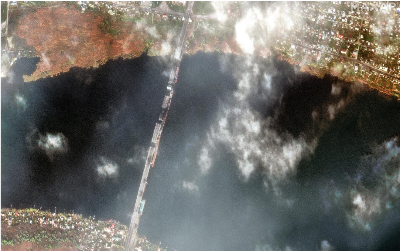
Overview of the damage to the Antonivsky Bridge on November 11. Source: Satellite image ©2022 Maxar Technologies
