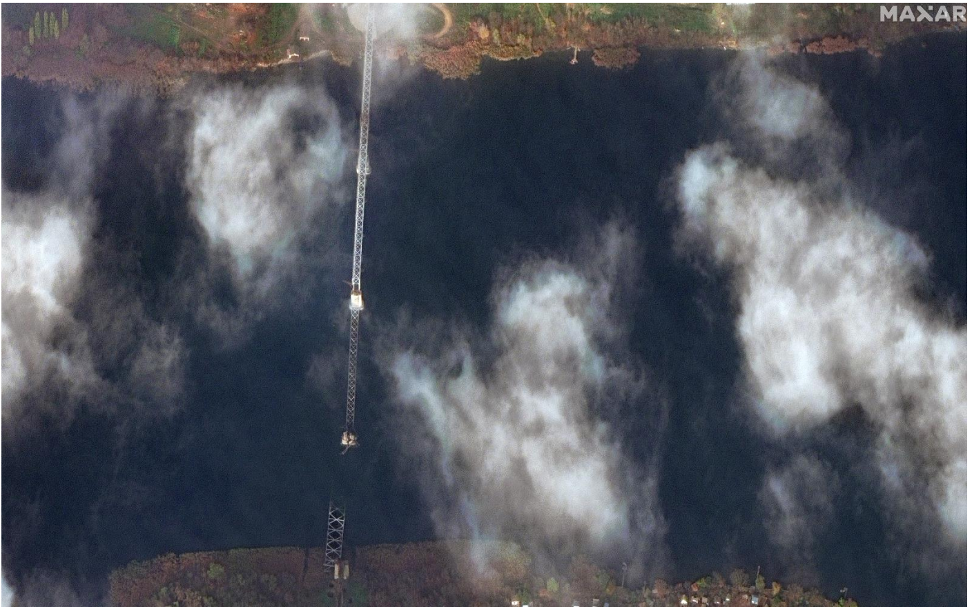
Overview of damage to the Antonivsky Railway Bridge on November 11. Source: Satellite image ©2022 Maxar Technologies
