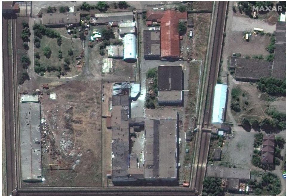
Overview of damaged buildings in Olenivka prisoner of war facility on July 30. Source: Maxar Technologies
